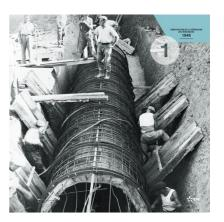
2 / Installation of the rotor for one of the generating units in the hydroelectric plant
